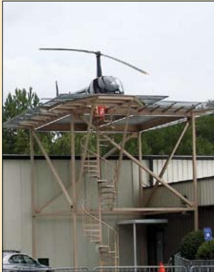
*The new Robinson-built helipad is supported by a free standing, 24-foot high steel platform.*
